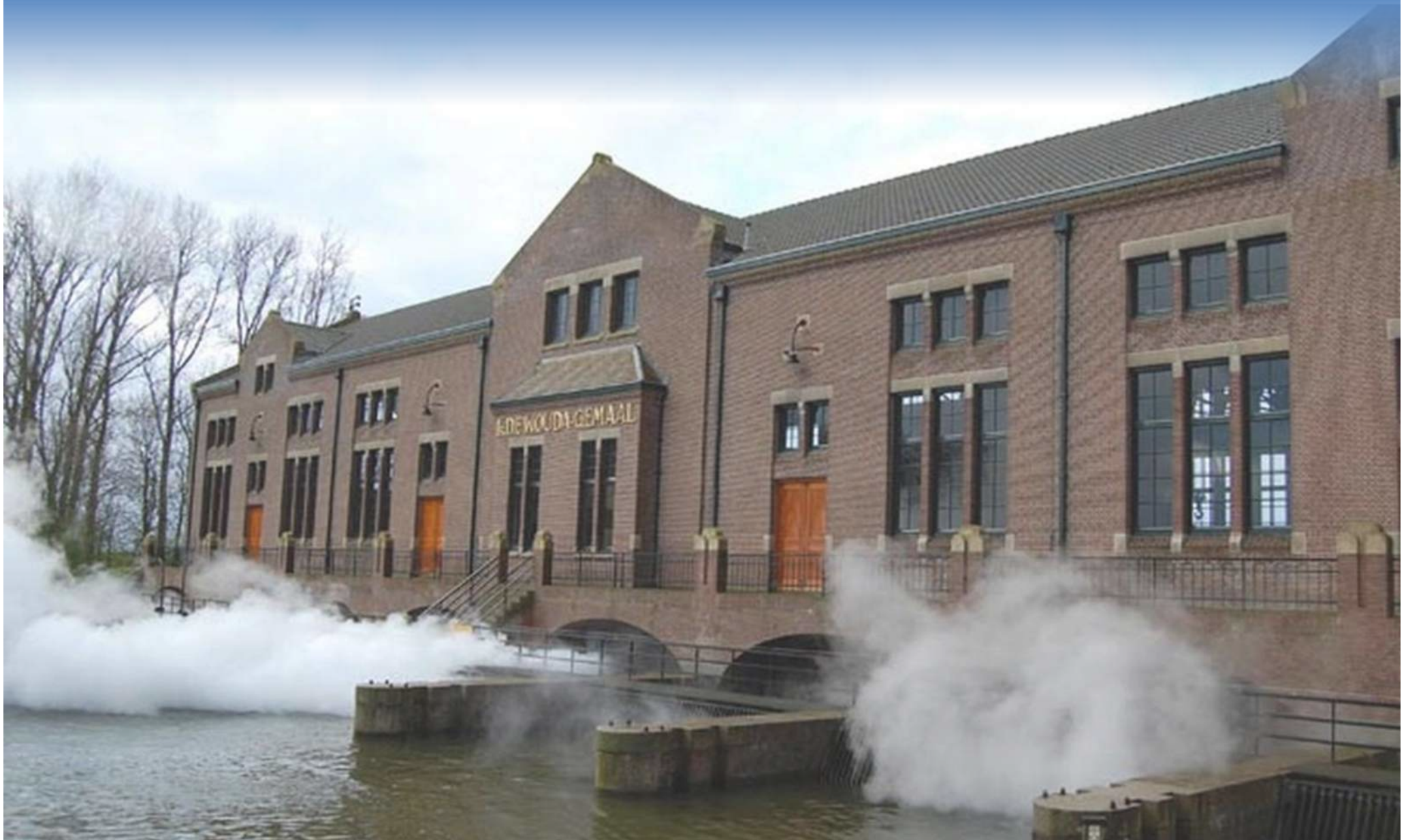
The D.F. Wouda steam pumping station (1920) at Lemmer, Friesland in full pumping action
