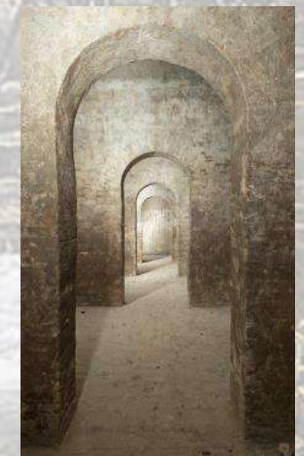
Water cellar under Lauriergracht 116 Amsterdam
