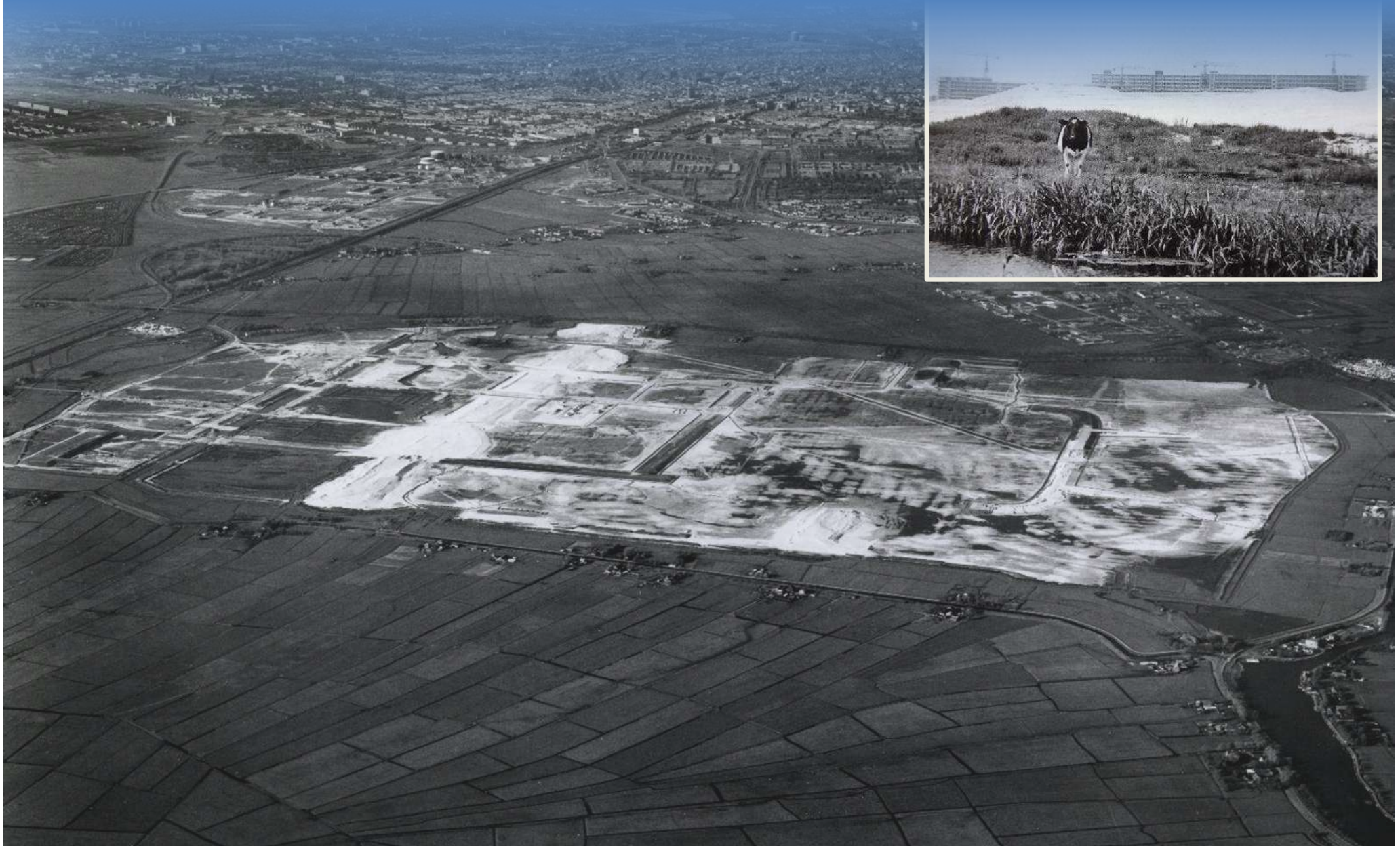
Raising the terrain for the Bijlmermeer housing estate of Amsterdam (1968) covering the peat landscape
